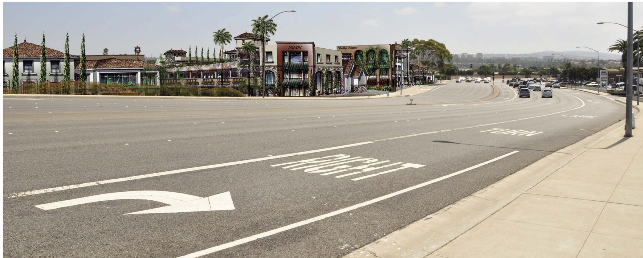
View Simulation #2 from the bridge along Pacific Coast Highway
