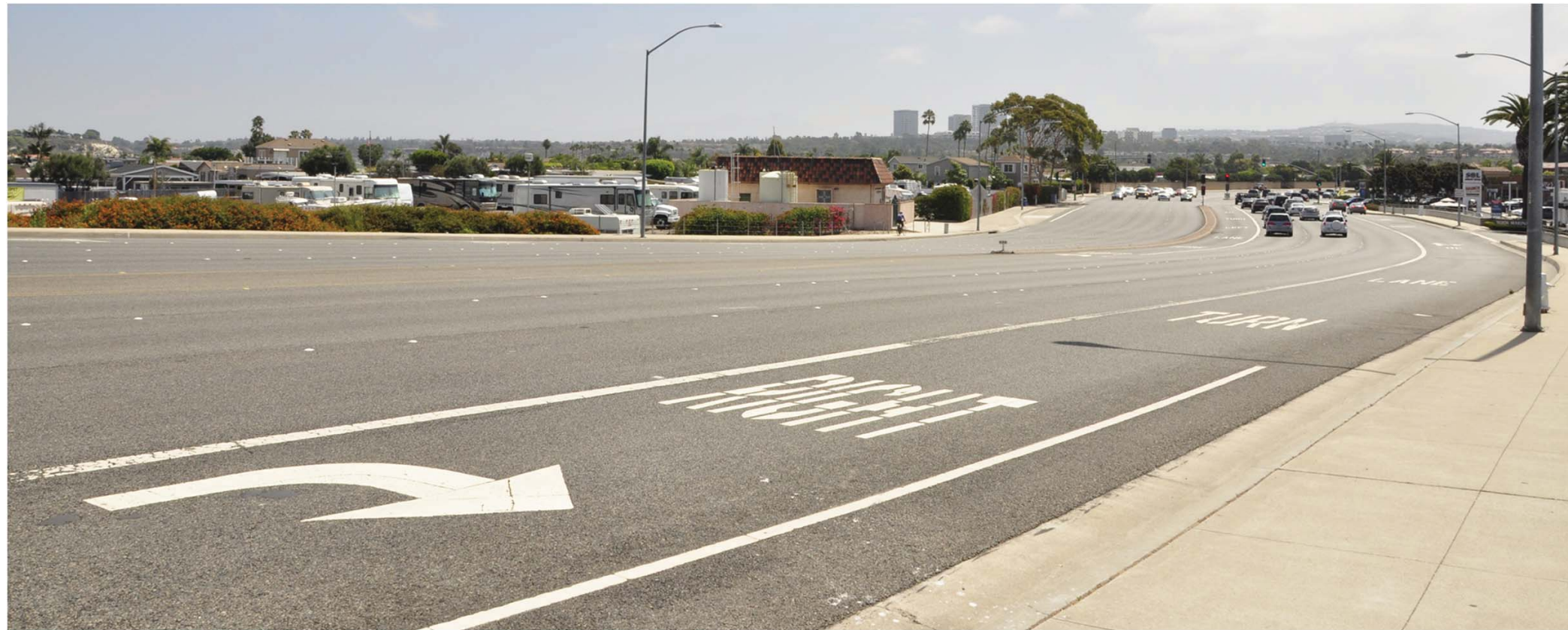
Site Photo from the bridge along Pacific Coast Highway
